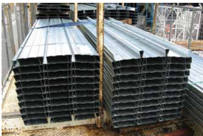
Step 1: Open BONDEK sheet bundles
