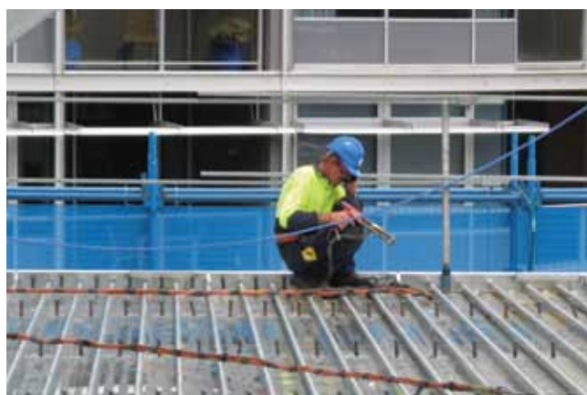
Step 4: Fix BONDEK sheets to steel beams if required
