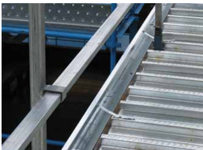
Step 5: Fix steel Edgeform
