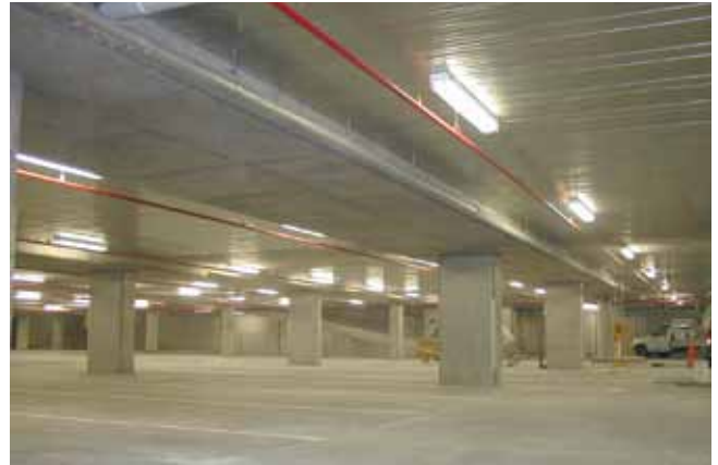
Step 9: Allow slab to cure and remove props
