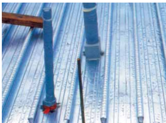
Step 6: Cut penetration
