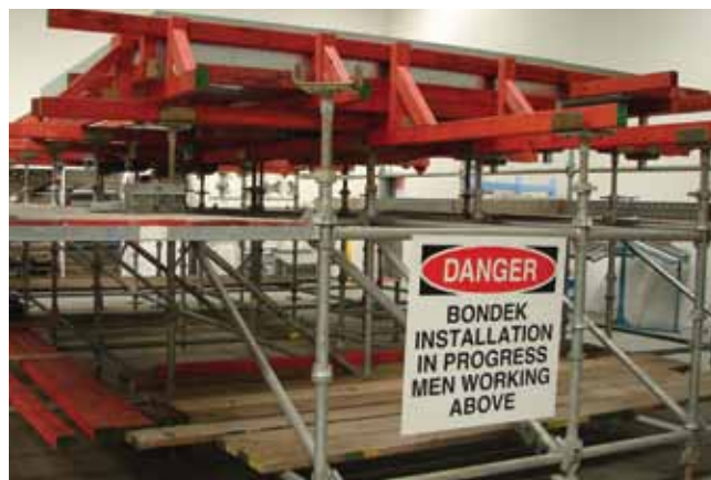
Step 2: Place props if required
