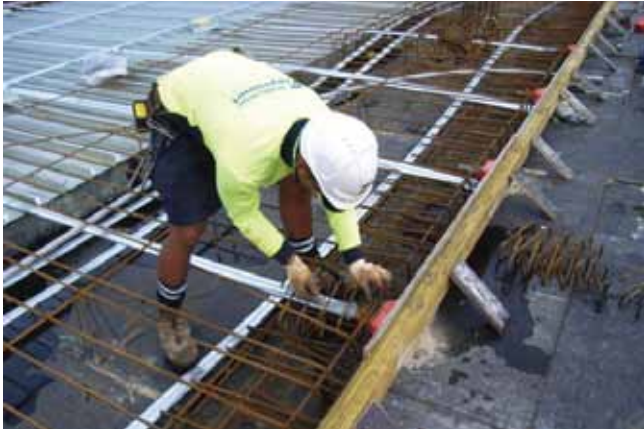
Step 7: Place reinforcement and post tensioning if required.
