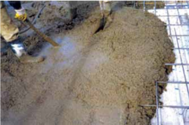
Step 8: Place concrete
