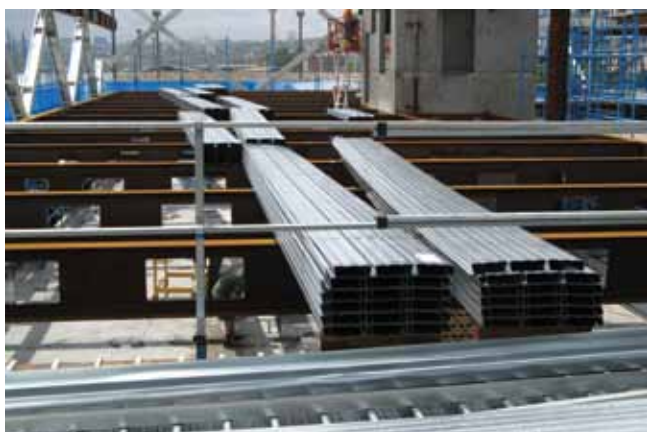
Step 3: Trim BONDEK sheets if required and place
