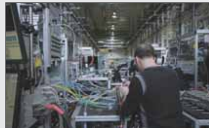
Ballard's 60,000 square foot test lab offers integrated data collection & reporting.
