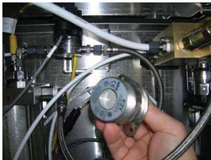
Figure 16 Combustible Gas Sensor Removed
