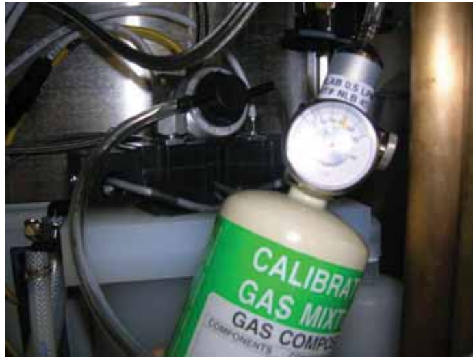
Figure 17 Calibration Hood installed on Combustible Gas Sensor
