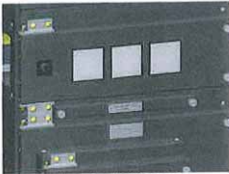
Upper test point access
