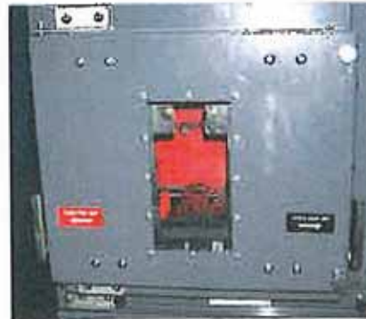
Circuit breaker closed and discharged
