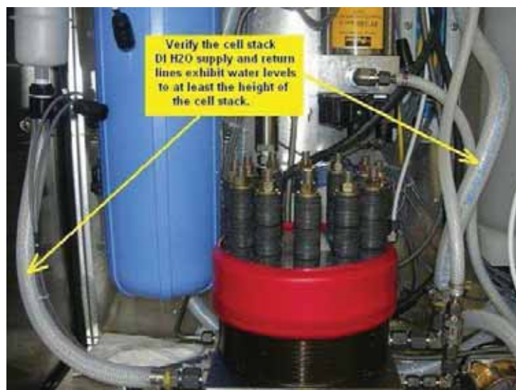
Figure 18 Cell Stack and Hydration Hoses
