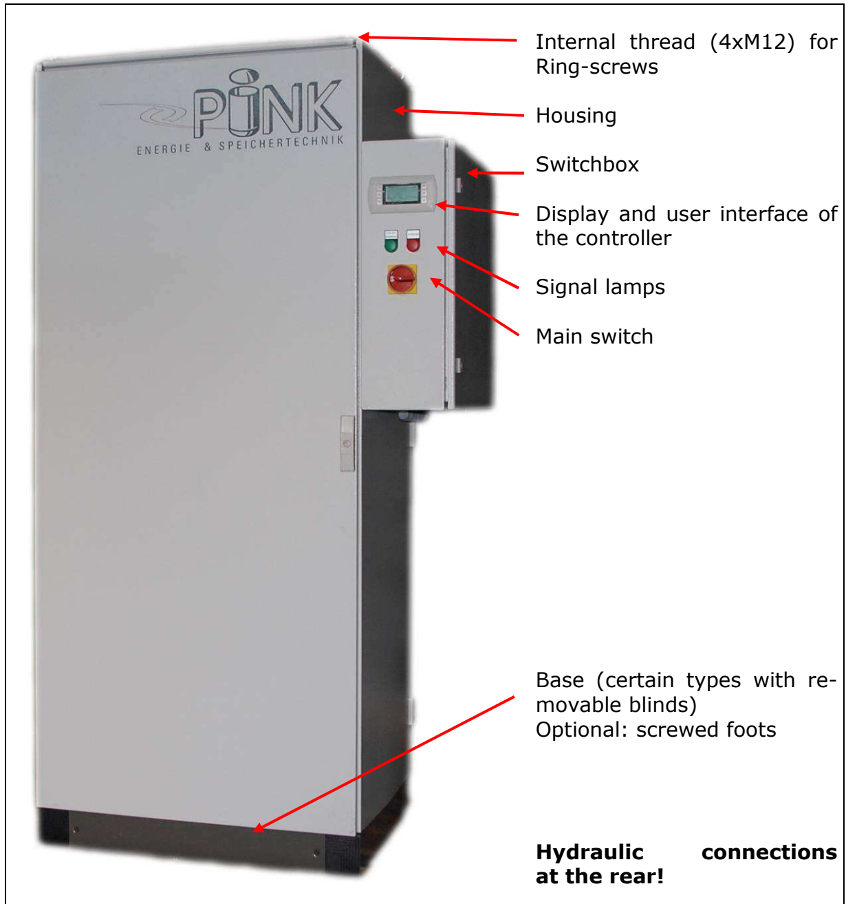
Figure 2: Components of the absorption chiller PC19
